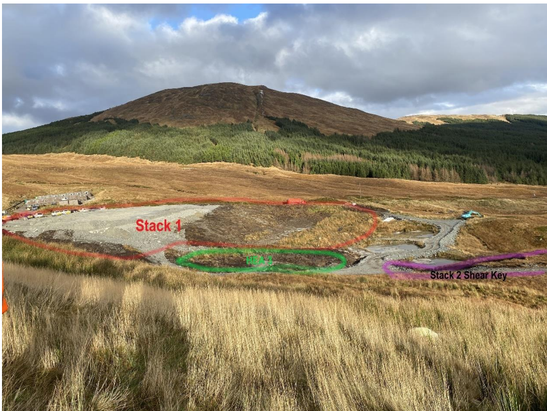
Image 2: Progress on Stacks 1 and 2 (November 2022)
