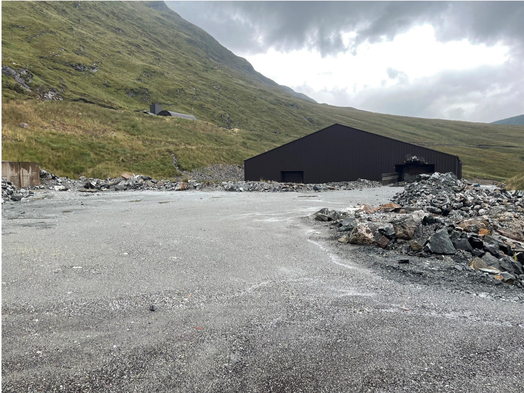
ROM Pad and Processing Shed, under Care & Maintenance
